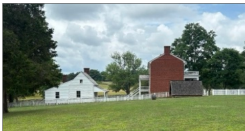
McLean House, with slave quarters and kitchen in back
